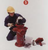
Remove the main valve assembly by pulling up and out on the upper stem
