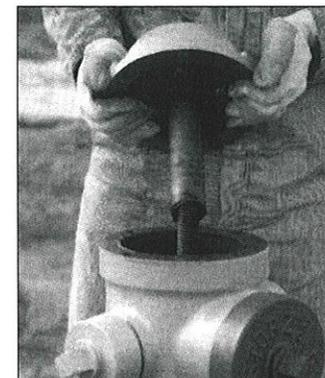
(3) For Bolt on, take out the four cap screws and remove body cap assembly by backing operating nut off of the stem.
