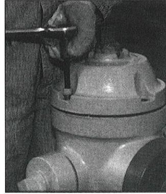
(2a) Shut off water at isolating valve. Open hydrant no more than two or three turns to relieve pressure. Remove the four cap screws.
