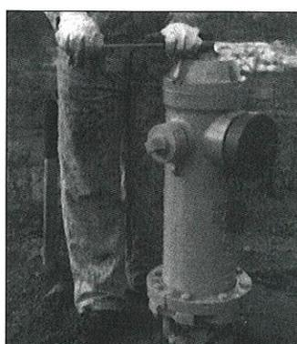
(7) Always operate hydrant after servicing. 18 turns  $\pm$  1 turn is standard.
