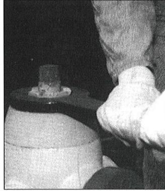
(2) Unscrew body cap anti-clockwise from the body, using a wrench on the top of the body cap. Remove body cap assembly by backing operating nut off of stem.
