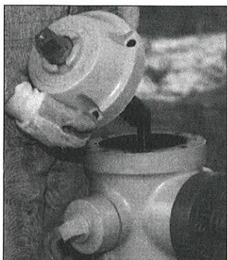
PLEASE NOTE: Oil hole screw should be removed to allow excess grease to escape.
