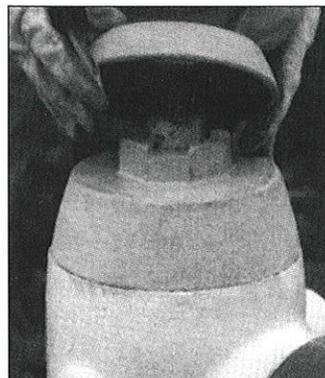
(1) Shut off the water at isolating valve. Take out body cap cover screws and remove cover.
